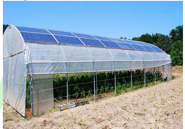
Fig. Solar greenhouse
