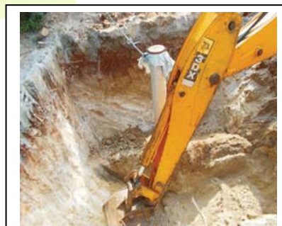
Fig-1 Recharge pits
