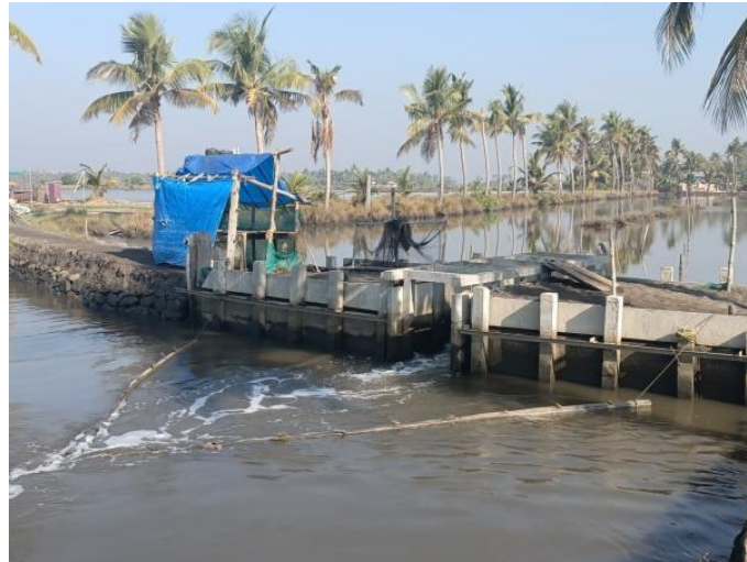
Fig.1 Sluice gate for controlling water flow in Pokkali Farm
