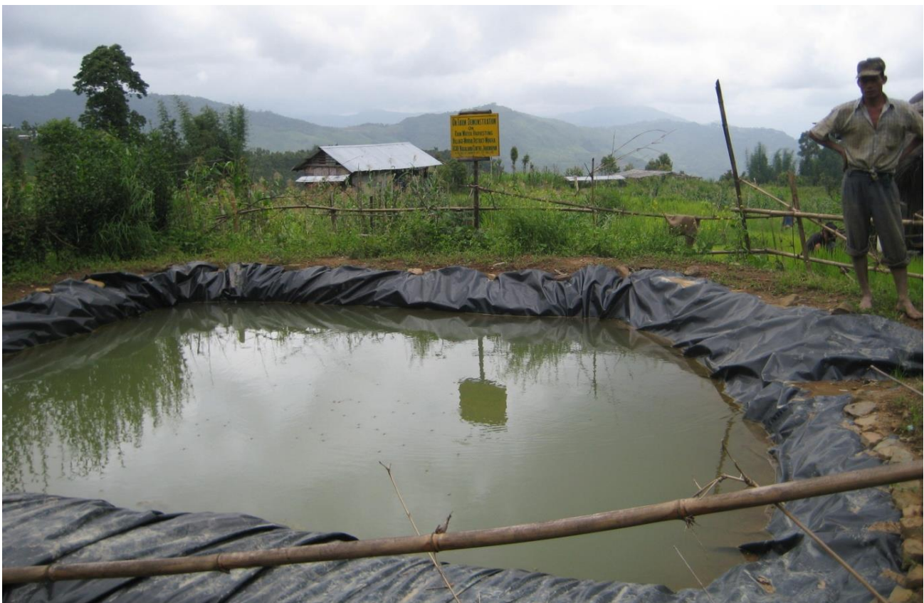
Jalkund constructed at Wokha village, Nagaland
