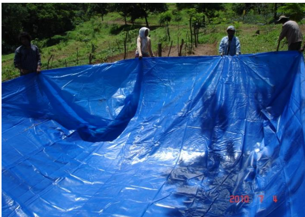
Lining of LDPE (250 \mu m) in the Jalkund at Langol, Manipur
