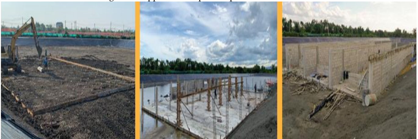
Pond reconstruction Slab construction with rebar posts Construction nearing completion
